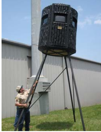
3. Tilt on two legs and remove fourth leg.
