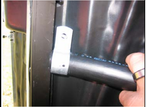
14. Penetrate predrilled hole in door frame with 1 1/4" Phillips head tapping screw and place EMT strap over screw.
