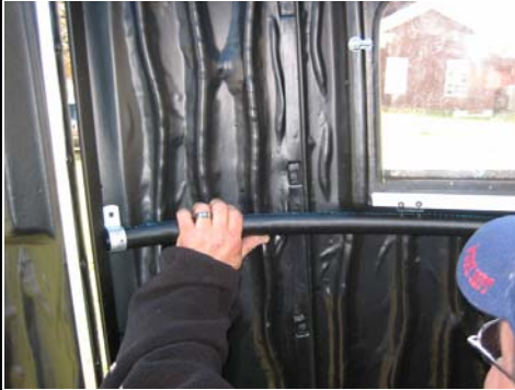
13. Start at door and work around using 1" EMT straps, screws and speed nuts.
